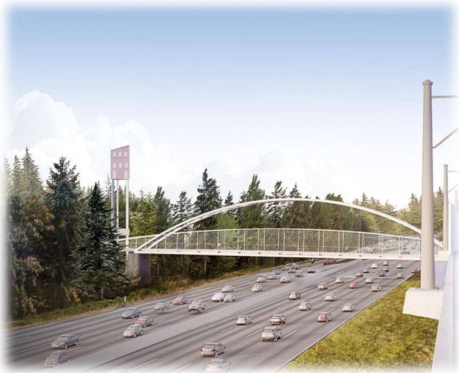
Figure 14 - Pedestrian Bridge (City of Shoreline, WA)
