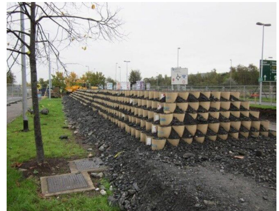
Figure 4.8. Structural framework of berm during construction process (FloodDefenseGroup).
