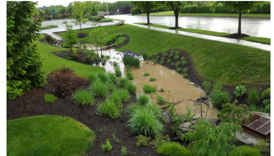
Figure 8.2 Bioswale as part of urban development (source: The Klausing Group).
