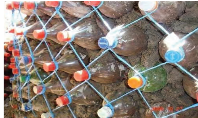
fig. 6.4. Cross section of bottles, cob, and string
