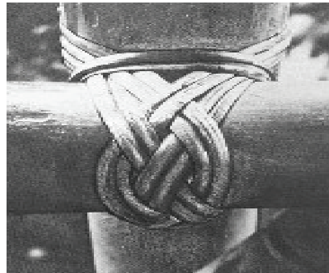
fig. 7.1. A simple bamboo lashing technique. Interlacing strips cut from green bamboo, the intersecting culms are interwoven with this lashing. When the bamboo lashing dries over the following weeks, the bond will get tighter.
