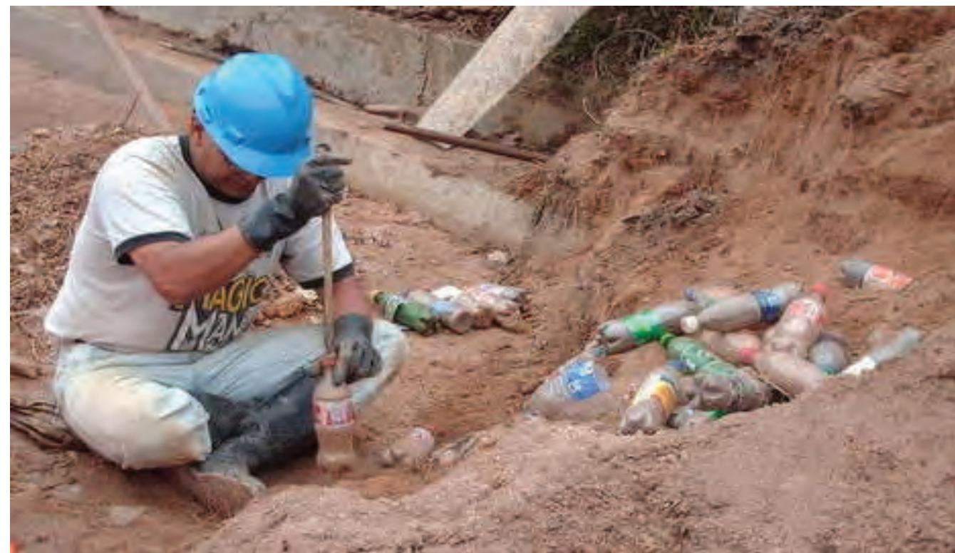
fig 6.6 Man filling bottles with sand
