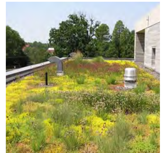
Example of intensive green roof
