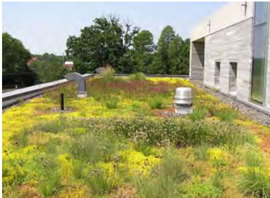
Example of green roof
