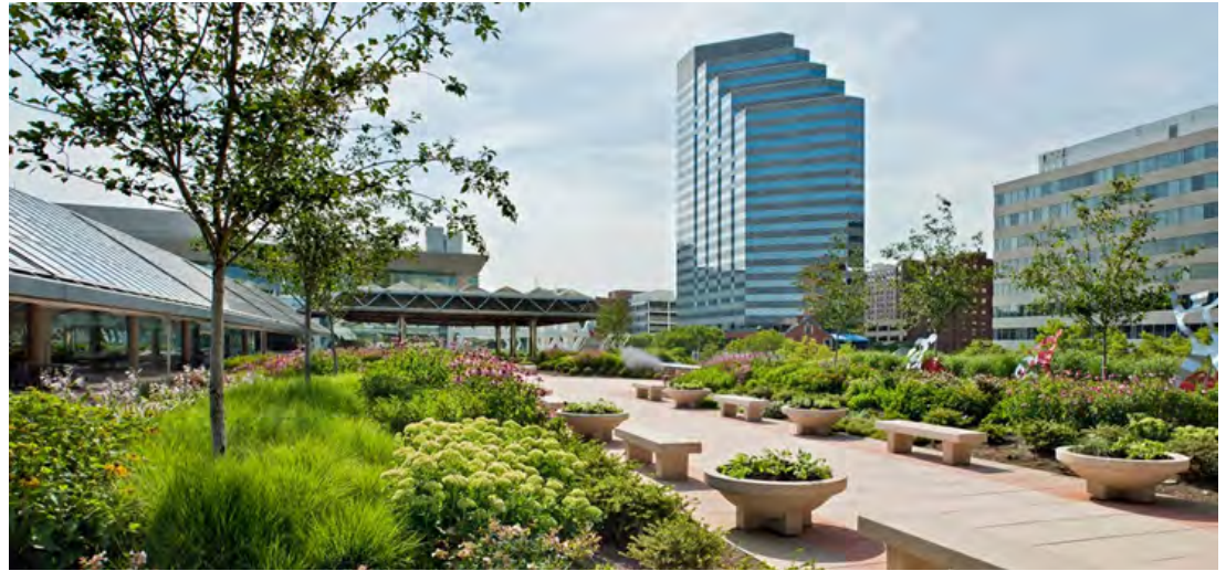
Example of extensive green roof
