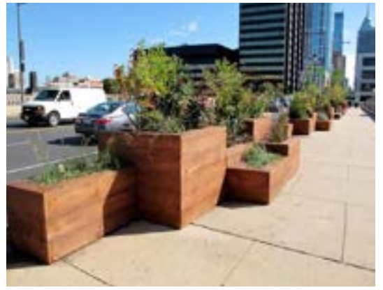
Figure 3.1.11. Raised planter boxes to separate cars from pedestrian traffic. Source
