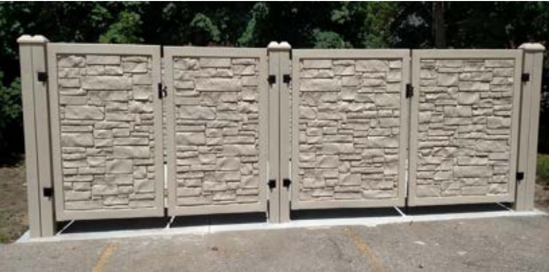
Figure 3.1.7. Faux stone dumpster coral. Source
