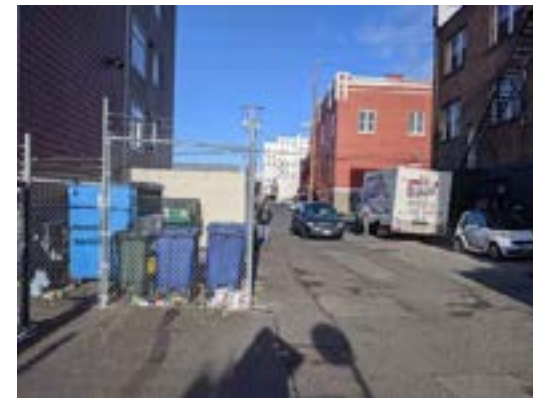
Figure 3.5.11: Site of where fenceimprovements should take place
