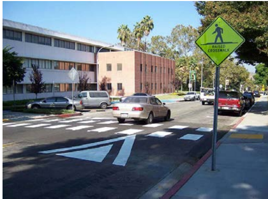
Figure 9.9 Raised crosswalk to provide safer crossing for children
