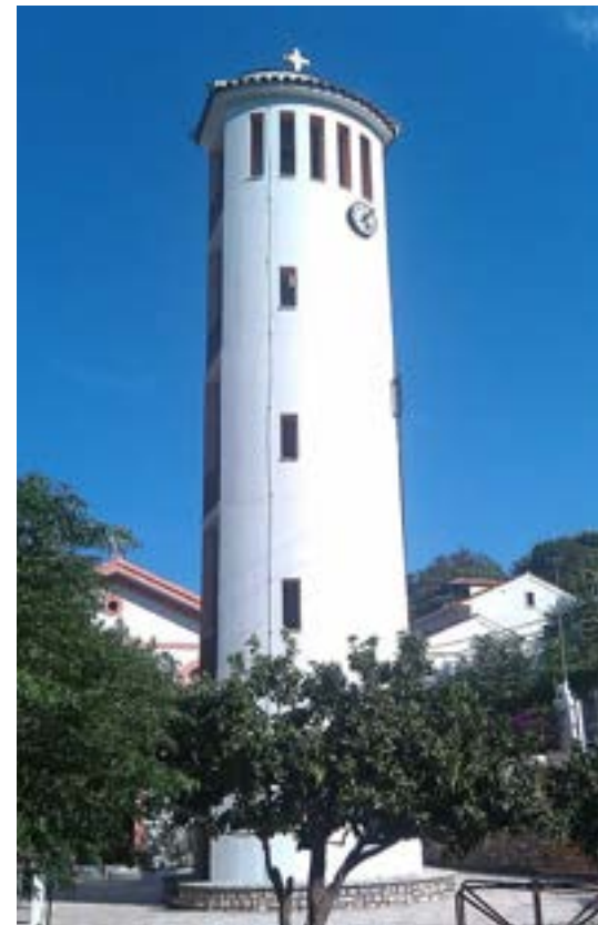
Exist bell tower, depicting modernism architectural style
