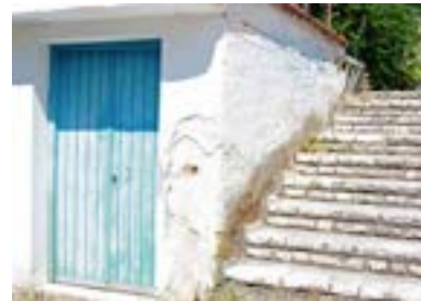
Node 3. A pedestrian path meets the Perdika hillside road.
