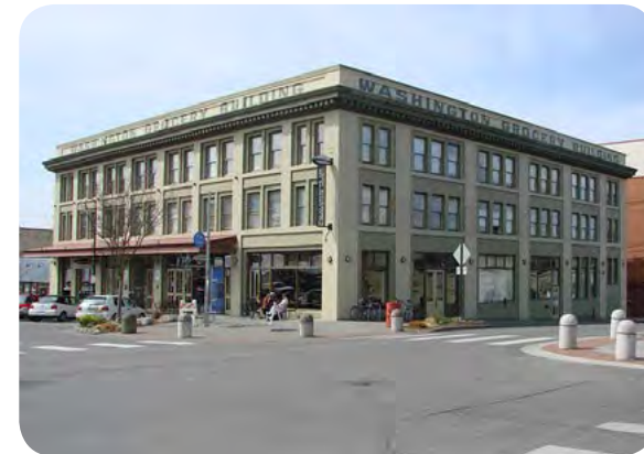
Washington Grocery Building 1133 Railroad Avenue, Bellingham WA 98225
