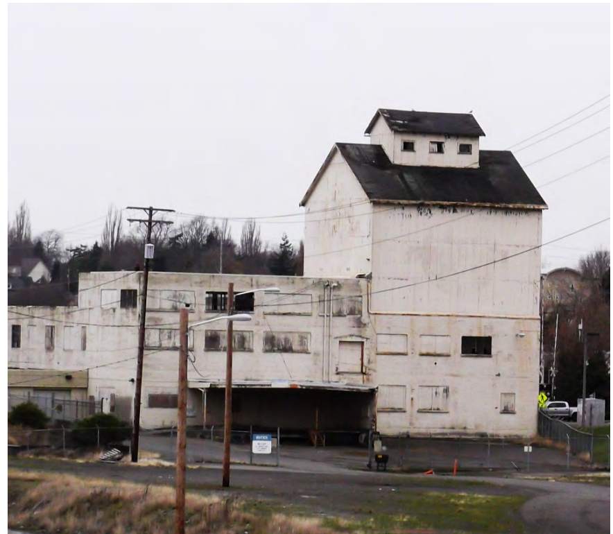
Fig. 1.2.5 Historic Granary Building
