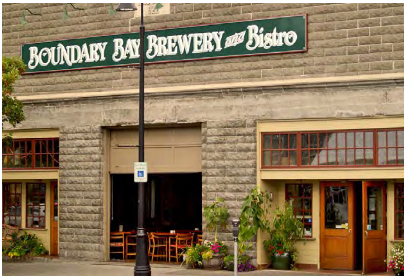
Figure 1.4.9: An existing building in Downtown Bellingham http://www.mgtmagazine.com
