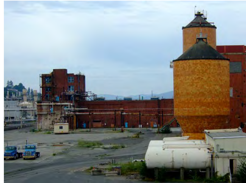
Figure 1.4.14: Existing waterfront buildings and their materials
