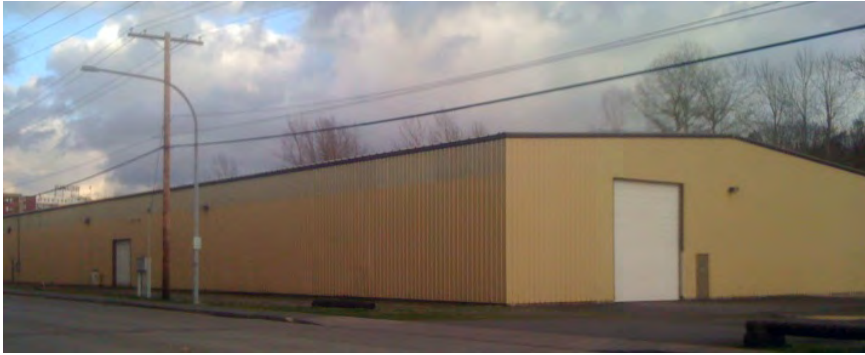
Figure 1.3.15 Existing Maritime Museum
