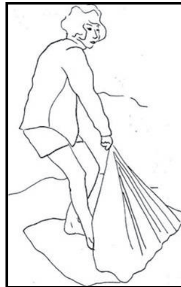
Stirring the cob mixture
