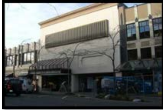
Figure 2.4: Example of black façade on Cornwall Avenue
