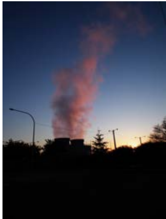
Encogen natural gas plant
