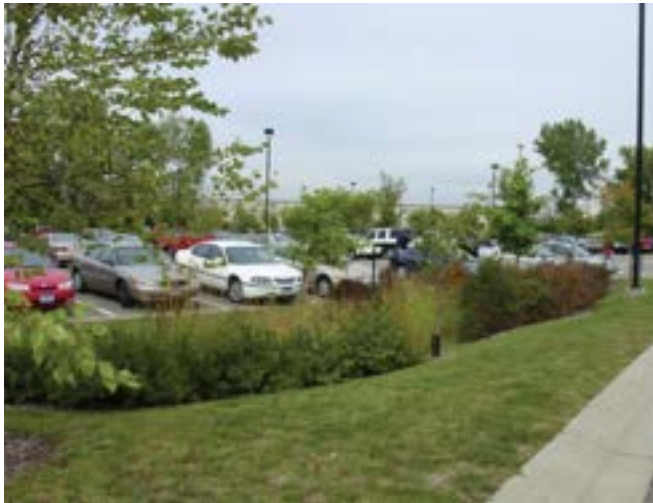
Figure 4. An example of a bioretention cell. Notice the vegetation in the landscaping of the cell, which could contribute to the aesthetic value of the pedestrian space near the proposed parking structure. Credit: USDA's Natural Resources Conservation Service ( www.ia.nrcs.usda.gov/features/urbanphotos.html ).
