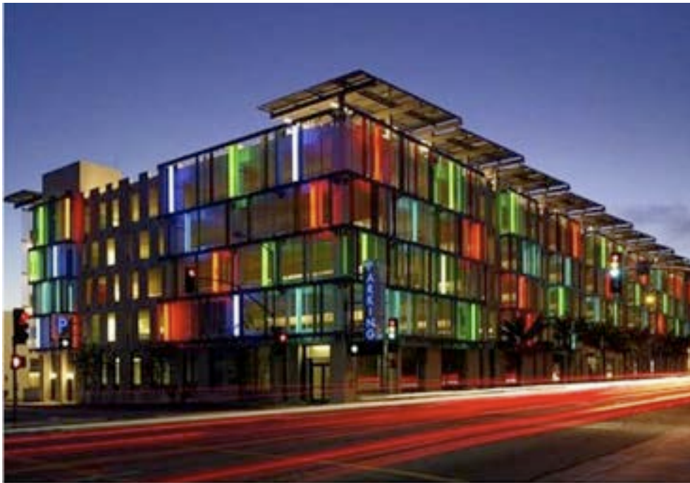
Figure 6.7: A LEED certified parking structure incorporating solar panels, Santa Monica, CA.
