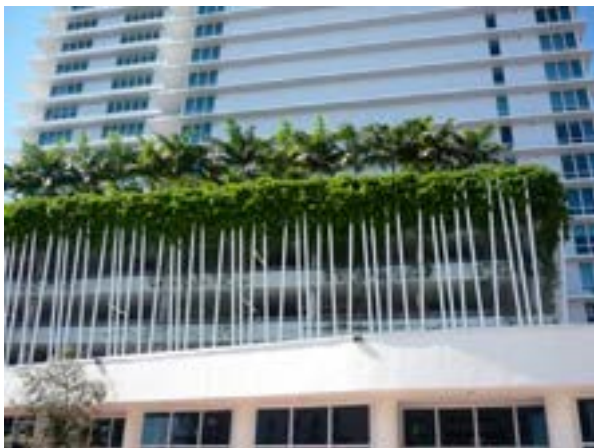
Figure 6.4: Image of a mixed-use parking structure with an urban garden in Miami, FL.
