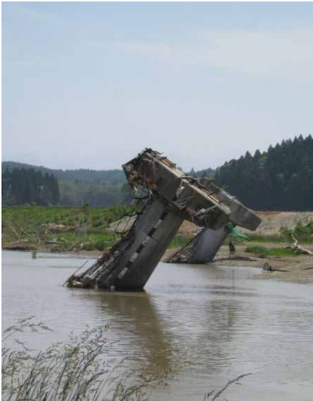
Figure 26. Tsunami waves following the 2011 Tohoku earthquake in Japan slammed into a pier supporting a rail bridge. The force of the tsunami waves washed away the bridge spans and heavily damaged the pier. Photo: Shideh Dashti.
