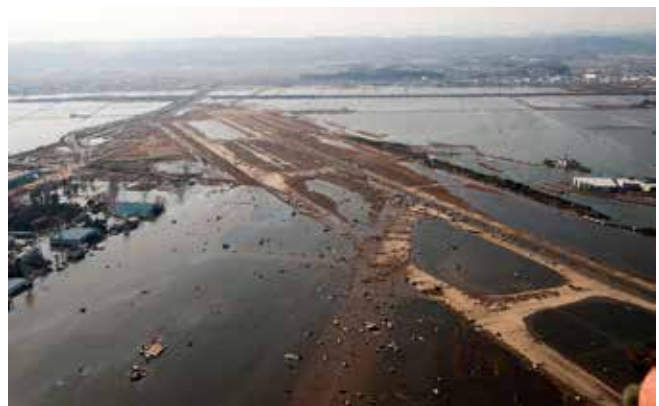
Figure 39. Tsunami waves resulting from the 2011 Tohoku earthquake, inundated the first floor and parts of the second floor of the terminal at Sendai Airport and littered runways and tarmac with debris. Photo: Staff Sgt. Samuel Morse, U.S. Air Force.
