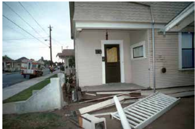
Figure 114. The 1989 Loma Prieta earthquake shifted this house over two feet off its foundation causing the structure to detach from the concrete stairway and collapsing all four shear walls. Photo: J.K Nakata, USGS.
