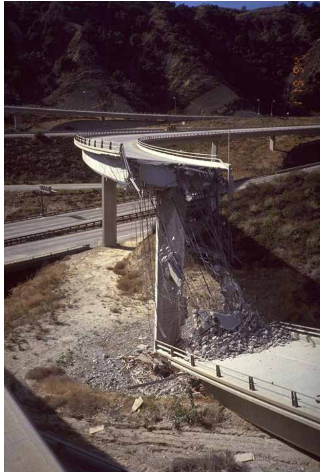
Figure 27. Following the 1994 M6.7 Northridge Earthquake in California, several freeway bridges such as this post-tensioned north to south connector ramp, completely collapsed. Heavily damaged and collapse of bridges that have not been seismically retrofitted may severely disrupt transportation and take years to demolish and rebuild. Photo: Guillermo Santana.
