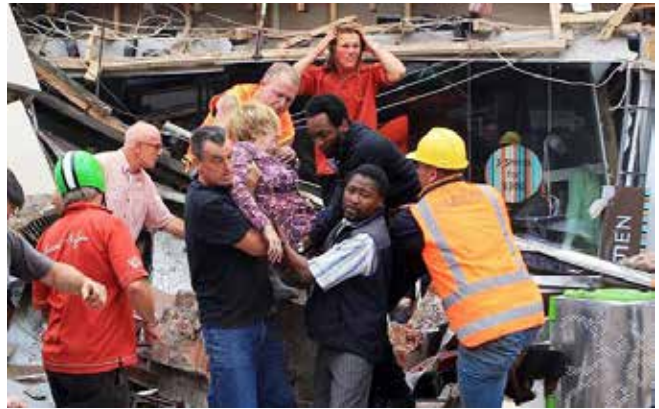
Figure 16. Rescue workers pull an injured woman from a collapsed building following the 2011 Christchurch, New Zealand earthquake. Photo: Reuters.
