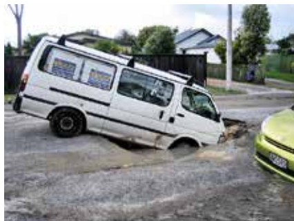
Figure 6. The 2011 Canterbury earthquake in New Zealand caused the loose sand and silt supporting the paved surfaces to liquefy and lose its ability to support this automobile. Liquefaction often results in uneven patterns of ground settlement. Photo: Martin Luff.
