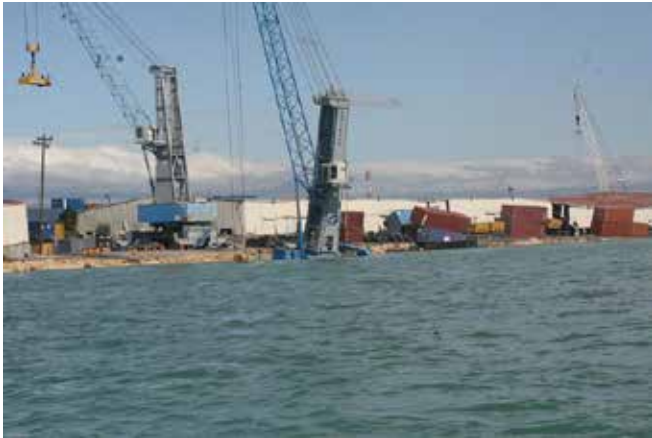
Figure 48. The 2010 Haitian earthquake caused medium damage to surrounding facilities, causing shipping containers to tumble and warehouses to derail. Ships were unable to deliver supplies and aid until repairs were made. Photo: U.S. Coast Guard.
