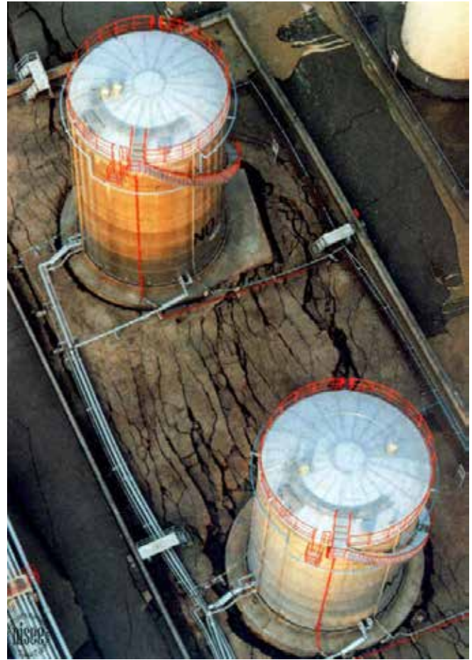
Figure 51. The 1996 M6.6 Kobe earthquake in Japan caused damage to pavement supporting tanks and other facilities. Some of Washington and Oregon's port fuel facilities, such as fuel tanks and terminals, are situated on liquefiable soil. These facilities could spill or rupture during the earthquake, posing serious fire and explosion threats. Photo: HITRAC.
