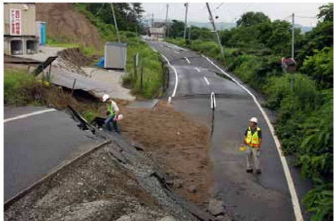
Figure 21. The 2007 Niigata earthquake in Japan triggered landslides that took out portions of roads. Some critical roadways in Oregon and Washington were built atop preexisting landslides, which could be triggered again during the earthquake. Source, CREW.
