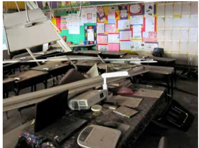
Figure 88. The 2010 Baja California M7.2 earthquake caused extensive damage to Jefferson Elementary School in Calexico, California, such that the school was closed for the remainder of the semester. Interior damage and fallen items could injure or kill students and faculty. Photo: Kelly B. Hutson.
